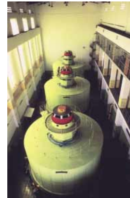
Turbines turn generators at a hydroelectric power plant. (Luis Casanueva/The Image Bank)
