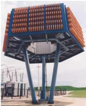
This bank of capacitors stores electrical energy for use in the particle accelerator at Fermilab, located outside Chicago. Because the electric utility company cannot provide a large enough burst of energy to operate the equipment, these capacitors are slowly charged up, and then the energy is rapidly “dumped” into the accelerator. In this sense, the setup is much like a fire-protection water tank on top of a building. The tank collects water and stores it for situations in which a lot of water is needed in a short time.
