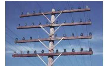
Electrical insulators on telephone poles are often made of glass because of its low electrical conductivity.
