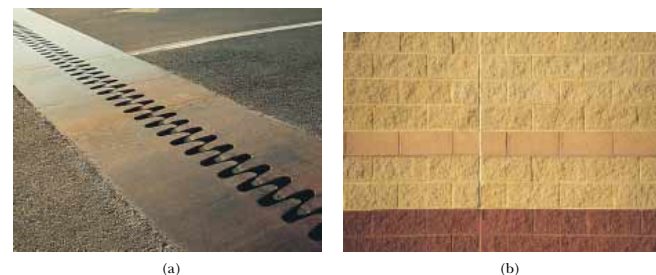
Figure 19.6 (a) Thermal-expansion joints are used to separate sections of roadways on bridges. Without these joints, the surfaces would buckle due to thermal expansion on very hot days or crack due to contraction on very cold days. (b) The long, vertical joint is filled with a soft material that allows the wall to expand and contract as the temperature of the bricks changes.
